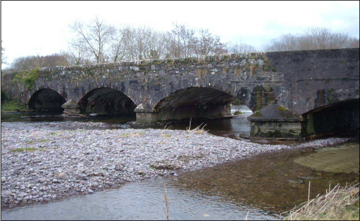
Plate 1: Bridge 111, Ballymakeera Bridge on the River Sullane
