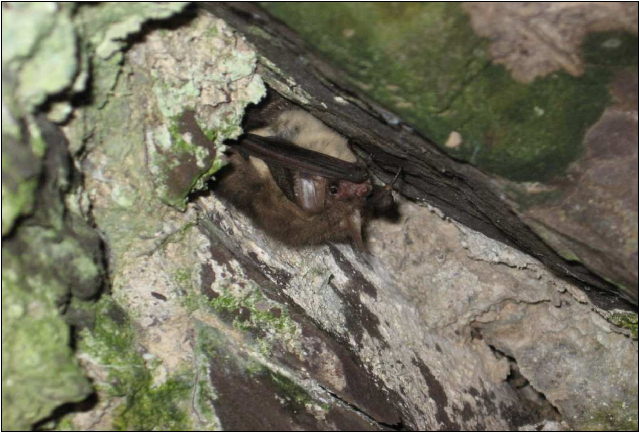
Plate 3: Brown long-eared bat using a crevice in a masonry bridge as a roost
